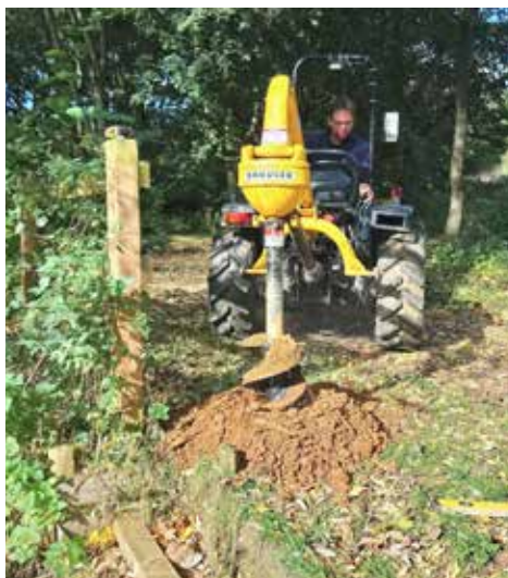
Ranger Andy digging post holes for the Folly Pond fence
